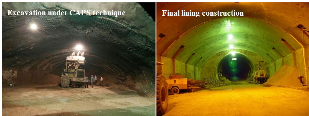
Fig. 5 Mellat single-deck station (N2 Station) of Tehran metro line 2 using CAPS method for the first time
